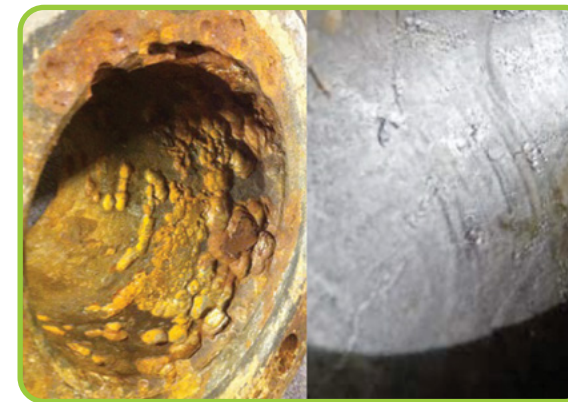
Typical Microbiological Influenced Corrosion damage to spool (left) vs. DragX™ application after 6 months (right)
