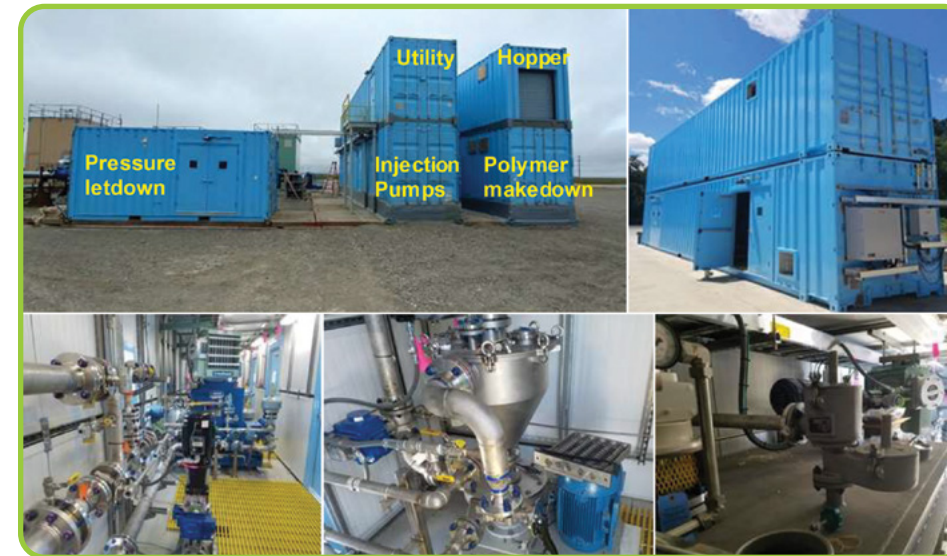
Polymer preparation equipment at NETL-supported field test on Alaska's North Slope.
